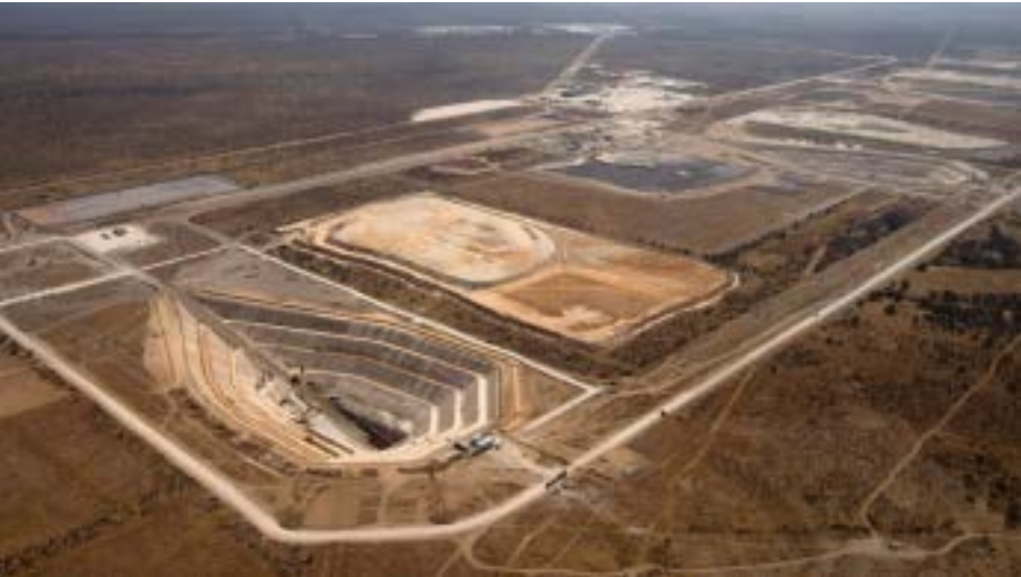
Figure 2-26: Infrastructure at Zone 5 of the Khoemacau mine, including two of the three boxcut portals that access underground operations.
